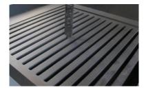
Turn the key 90° so that it is secured between the grooves of the grate. Now the grate can be lifted up with the door handle.
